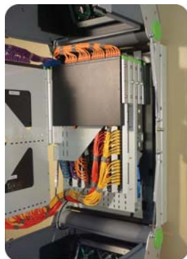
Vertiblade brackets provide full access to each piece of equipment.
