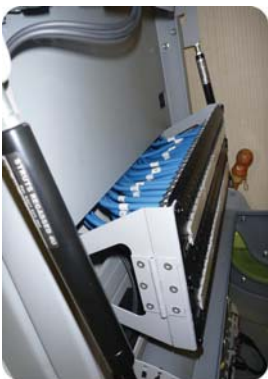
2055-CAT6 adapter hinged bracket provides required cable bend allowance.
